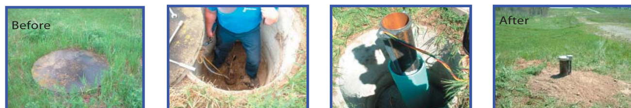
Upgrading a well pit to protect groundwater resources from surface water contamination.
