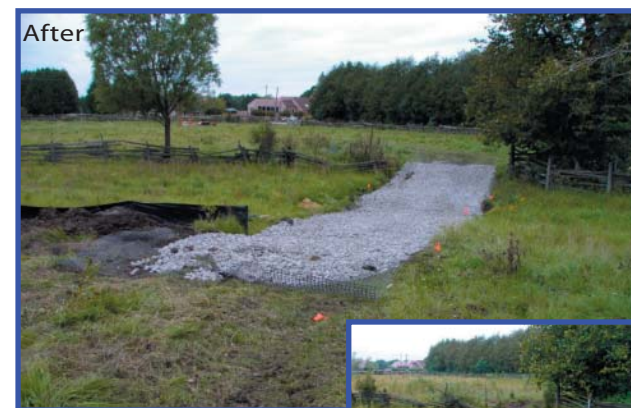
Before and after pictures of a livestock creek crossing.
