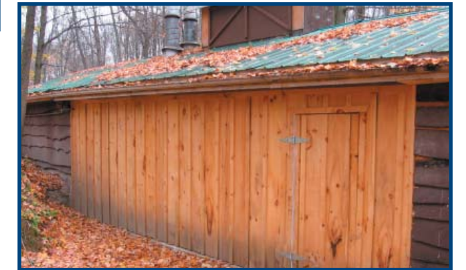
Sugar Shack Gets New Wall. Volunteers from the Joint Apprenticeship and Training Program (sponsored by the Carpenter's Local Union 27) completed repairs to the evaporator building at Purple Woods Conservation Area.
