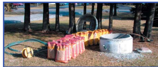
Bags of bentonite are used to decommission an unused well.
