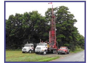
Borehole Drilling Rig.
