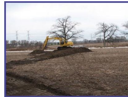
New trail construction at Bowmanville/ Westside Marshes.
