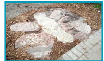
The new butterfly custom stone walkway.
