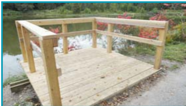
The completed viewing platform at Devil's Den pond.
