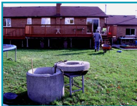
A well prior to receiving an upgrade.
