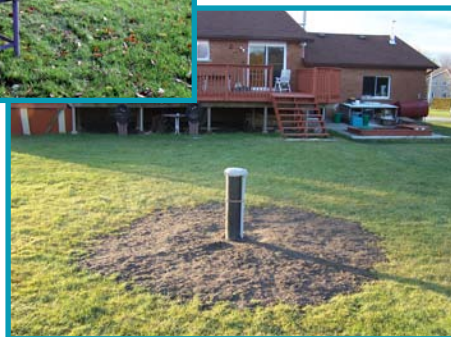
A well after the upgrade.
