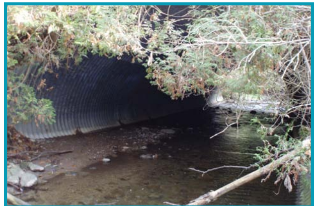
One of the culverts of the Lynde Creek Watershed.
