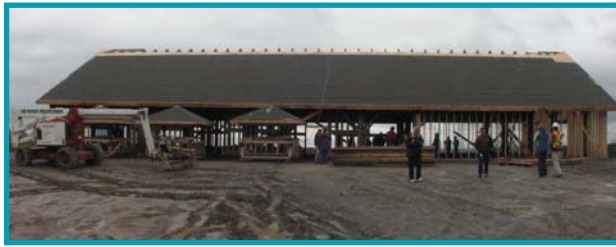
Purple Woods Conservation Area Heritage Hall under construction.
