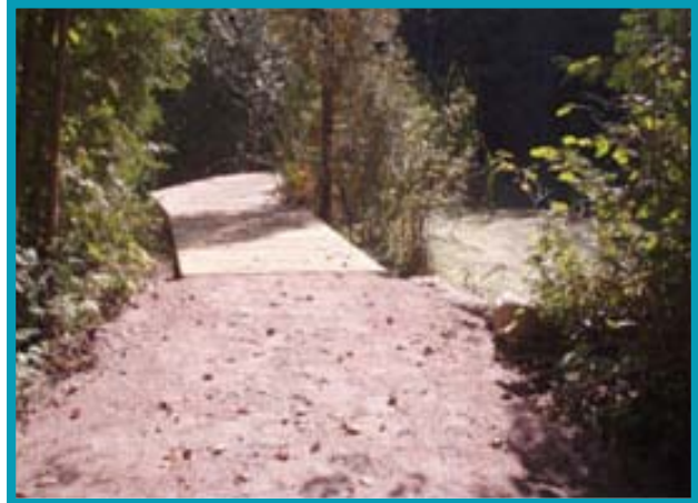
The new granite screenings.
