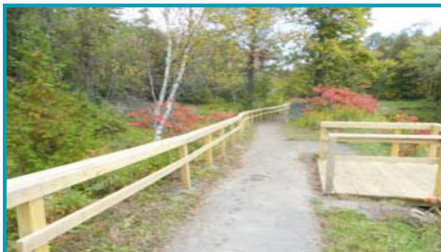
The new cedar safety railing installed by CLOCA staff around the pond.
