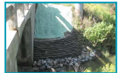
The new Envirolok system installed by CLOCA staff on Taunton Road.
