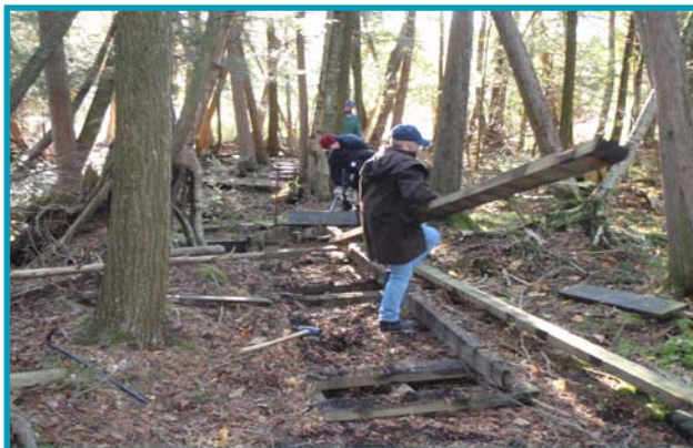
Volunteers decommissioning the boardwalk.
