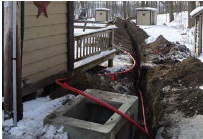
In preparation of a new maple syrup evaporator, the Sugar Shack underwent extensive renovations including a new hydro line from Coates Road.
