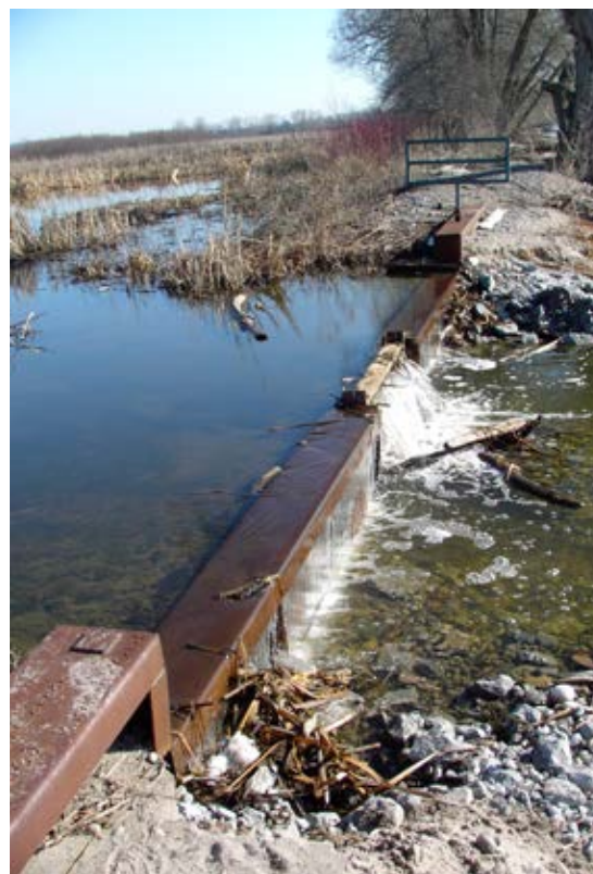
Cranberry Marsh water control structure
