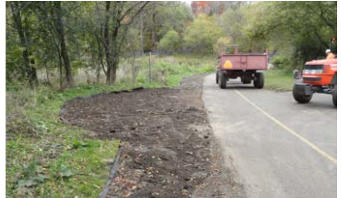
Working along the bike path.
