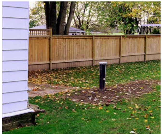
A well after being decommissioned by CLOCA staff.
