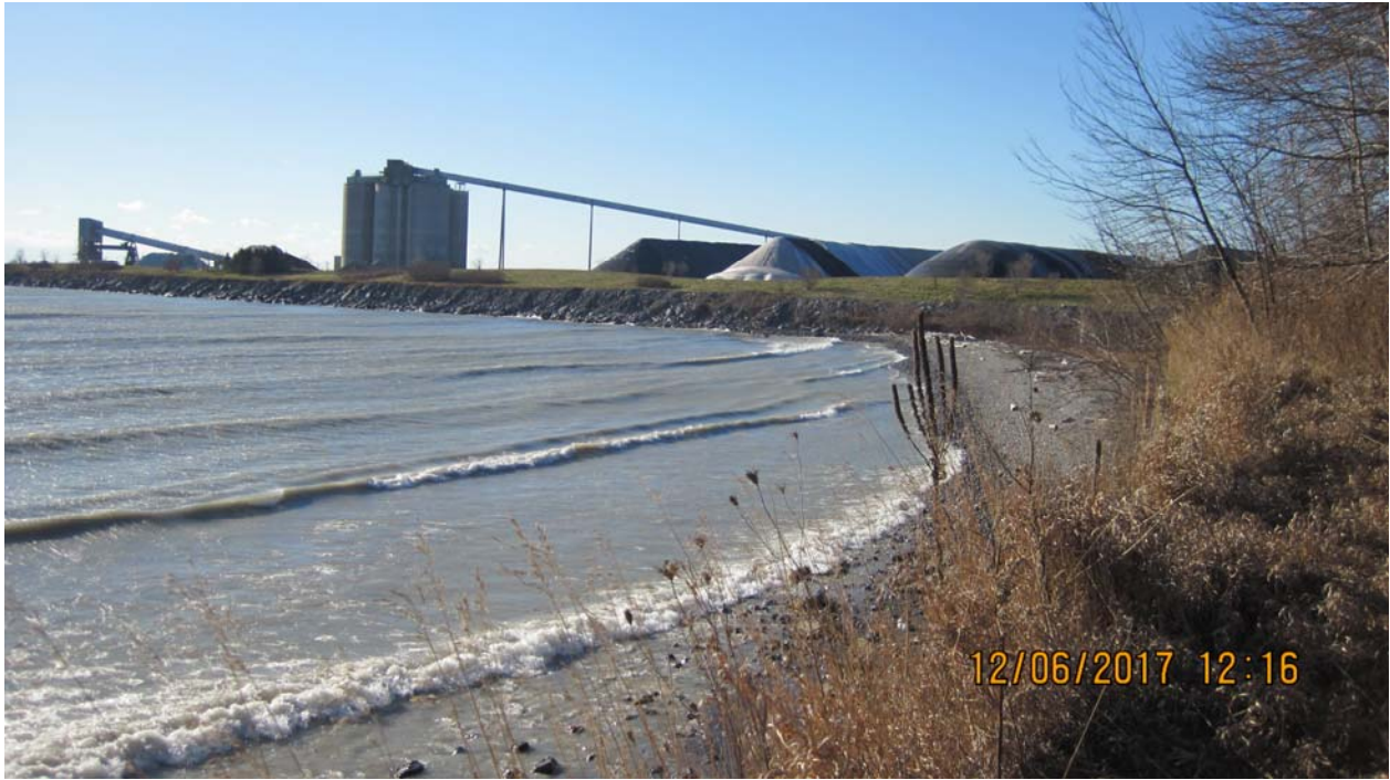
Figure 2.1: West end of study shoreline with fillet beach deposit on east side of St. Marys Cement
