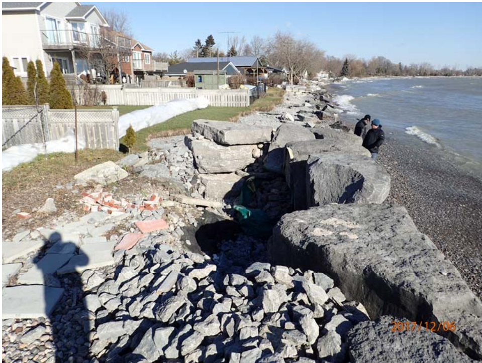
Figure 2.4: Armourstone protection at Cedar Crest Beach Road
