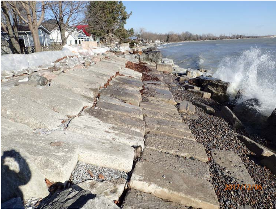
Figure 2.3: Concrete block revetment at Cedar Crest Beach Road
