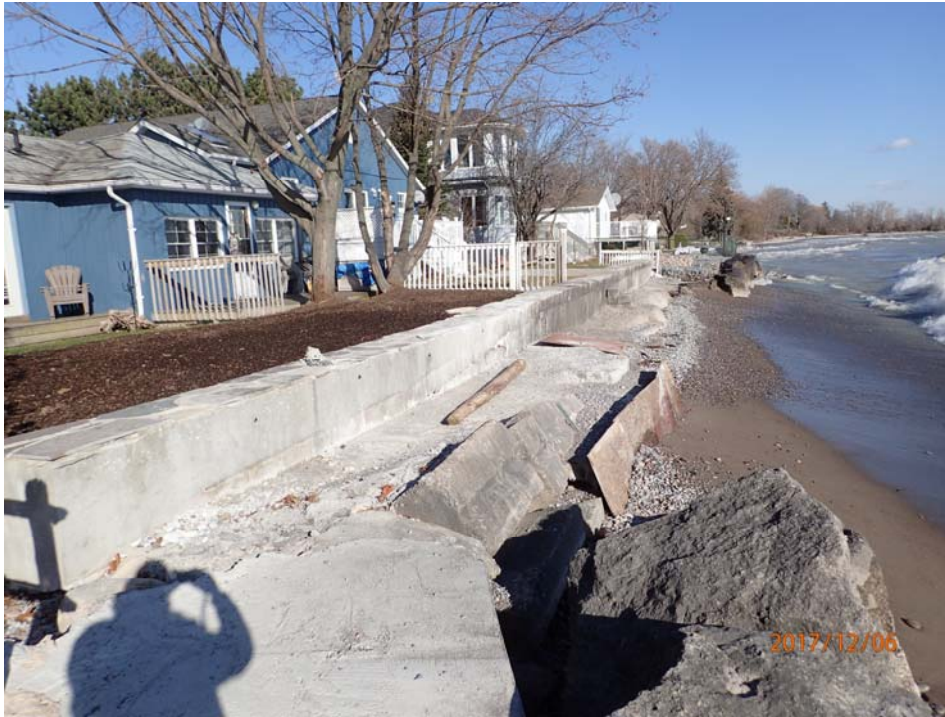
Figure 2.5: Concrete seawall at Cedar Crest Beach Road
