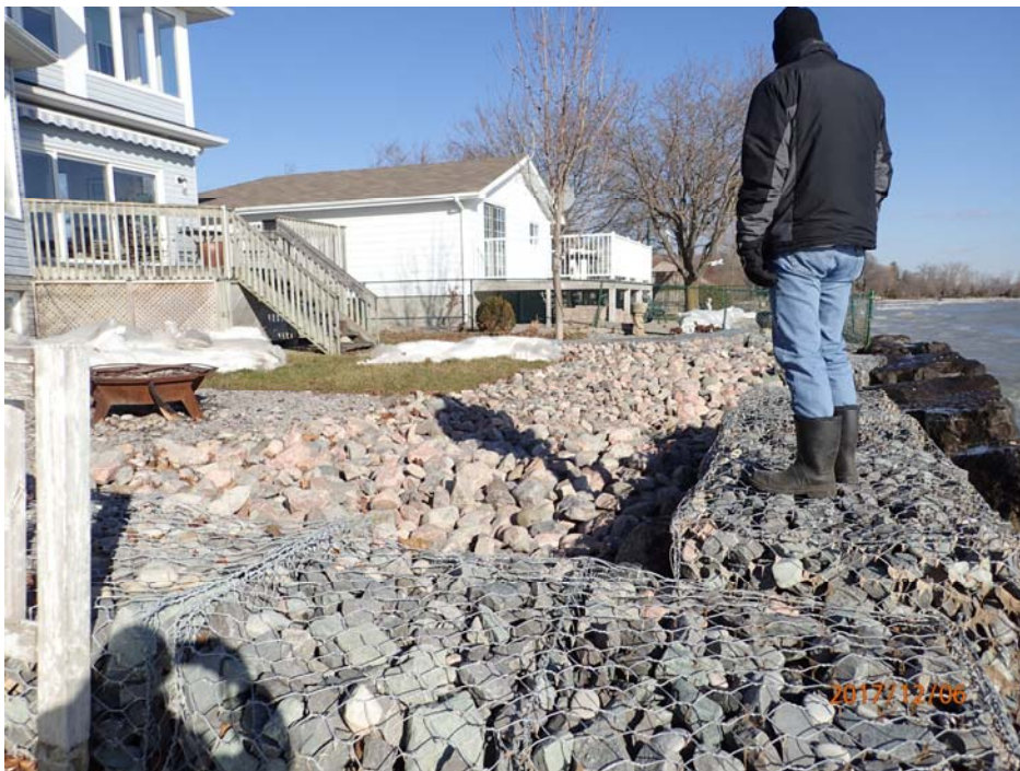
Figure 2.6: Gabion shore protection at Cedar Crest Beach Road
