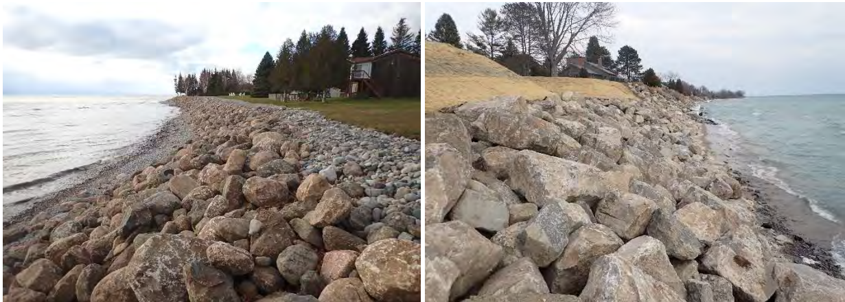
Figure 12 – Examples of conventional rubble-mound revetments with multiple layers of randomly placed field stone (left) and irregular armour stone (right).
