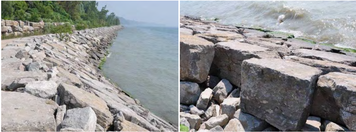
Figure 11 – Examples of single-layer, blocky armour stone revetments on Lake Ontario
