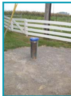
After well upgrade
