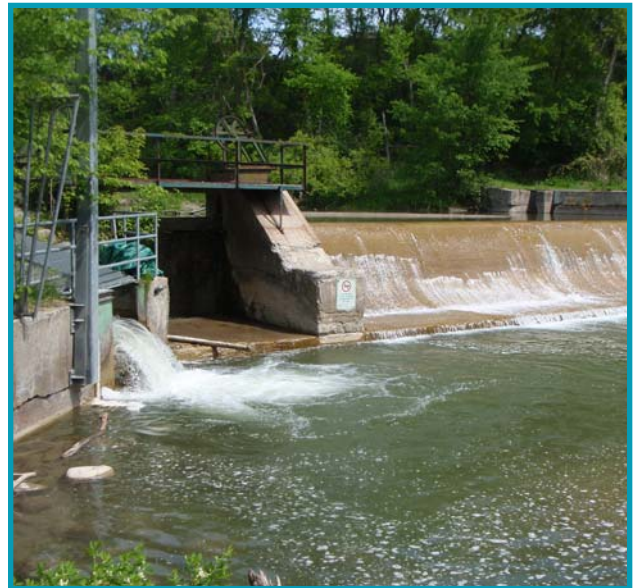
Plans are underway to incorporate a proper fish ladder into the Veyance Dam in Bowmanville to allow fish passage during migration.
