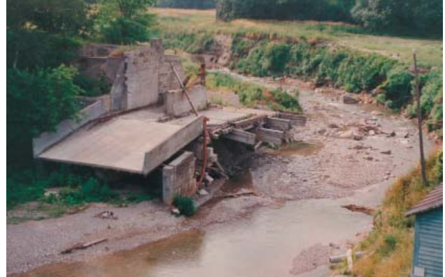
Van Stone Mill Dam after the flood in 1986.
