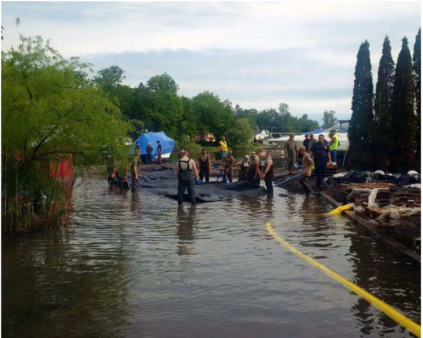
US Army National Guard members deploy a water-filled cofferdam by Sodus Point, New York, to help control Lake Ontario floodwaters. Credit: US Army National Guard
