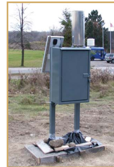
Precipitation water monitoring station.
