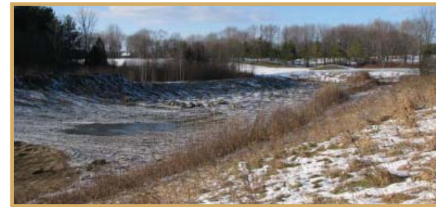
Almost complete, the wetland complex at Royal Ashburn covers 1.6 hectares (4 acres).
