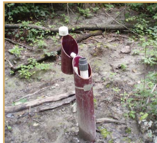
Drilling complete, the wellhead will be fitted with scientific equipment and added to the Provincial Groundwater Monitoring Network.
