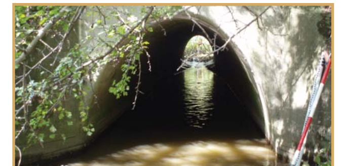
The first step in floodplain mapping is to survey all existing creek road crossings.
