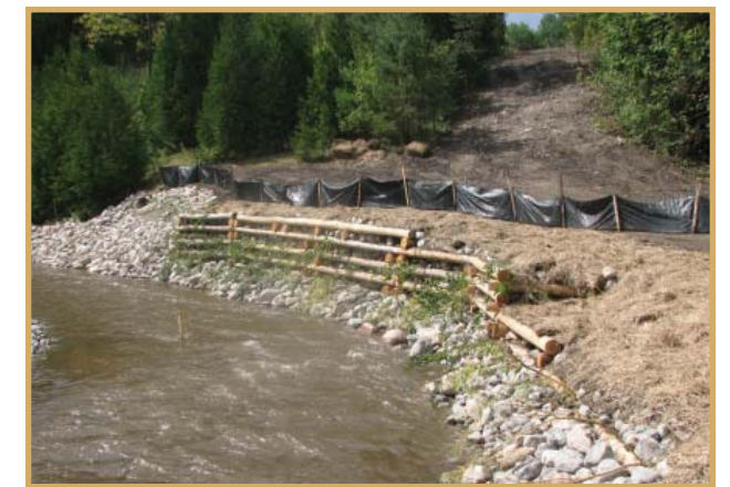
Bioengineering - A live crib wall is used to prevent streambank erosion on a local creek.
