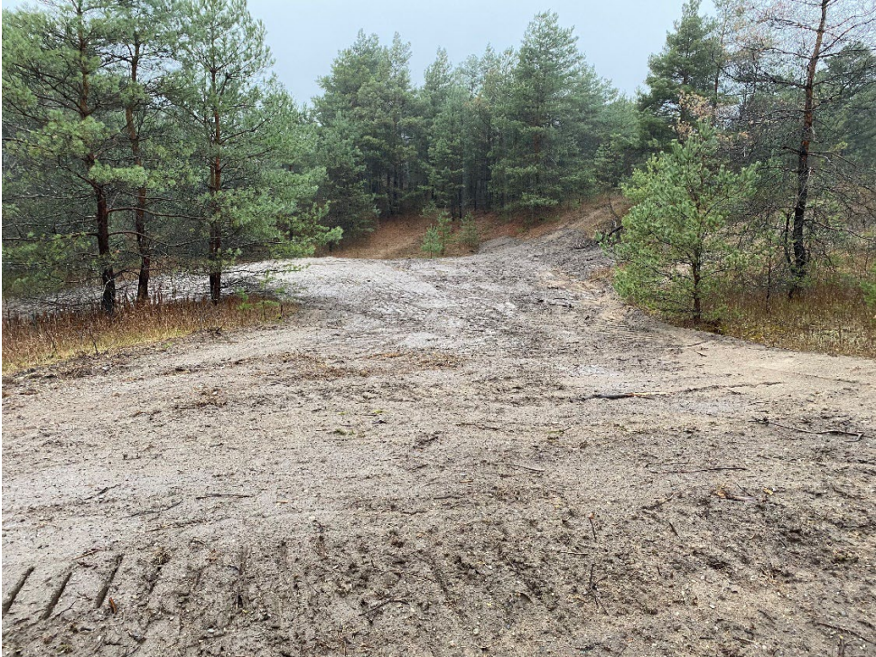
Photo 6, graded pit restoration area
