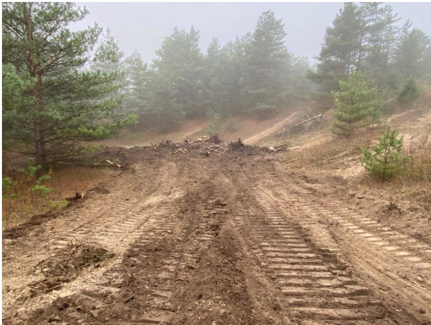
Photo 2; Surplus topsoil and woody material dumped and graded in abandoned pit area
