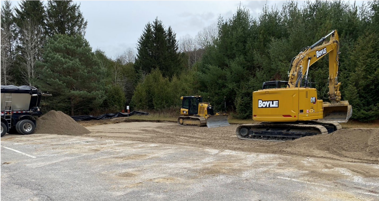
November 2022 – Granular B base compacted and Granular A arriving
