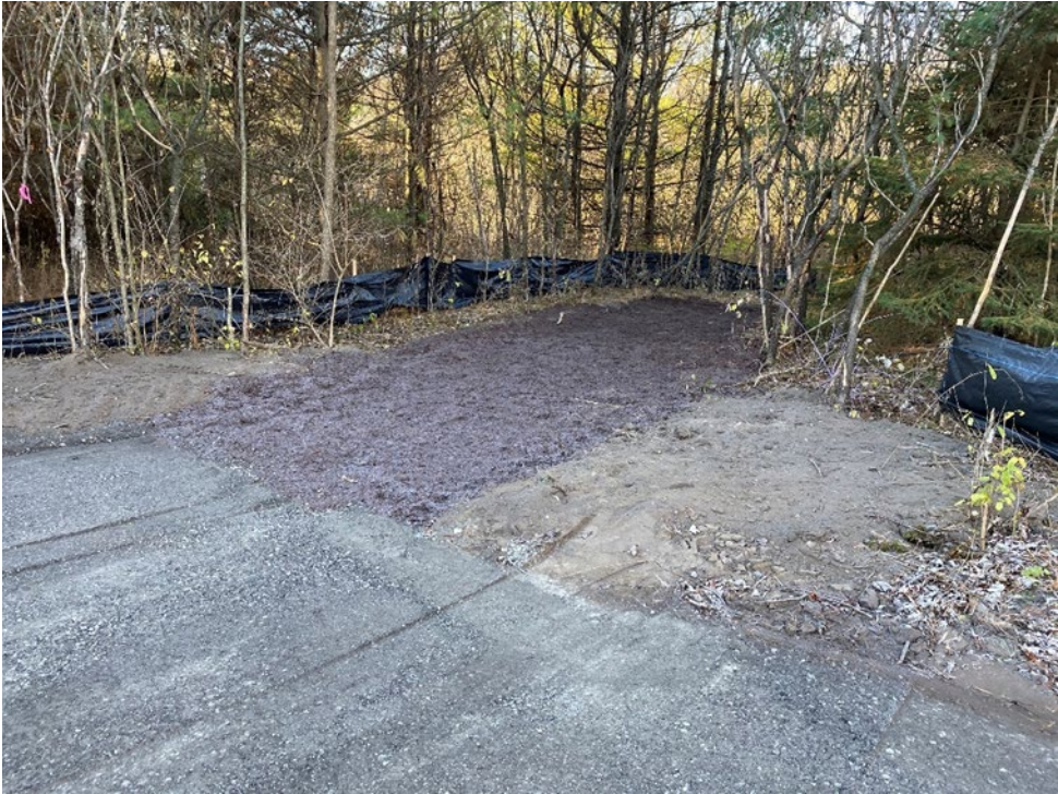
Photo 5 completed bioswale
