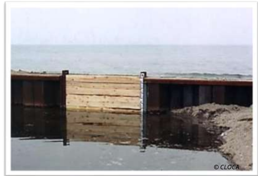
FIGURE 2: STOP LOG CONTROL STRUCTURE AT CRANBERRY MARSH.
