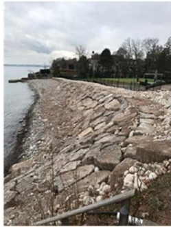
Figure 31 (Figure 3.4 from Baird Report) – Concept 4: Armourstone Revetment
