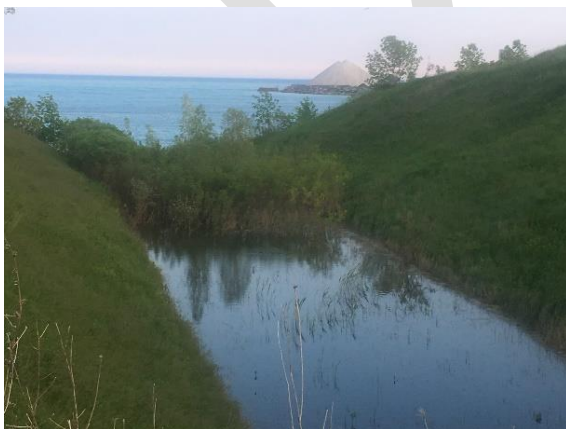
Drainage Channel - June 11, 2017
