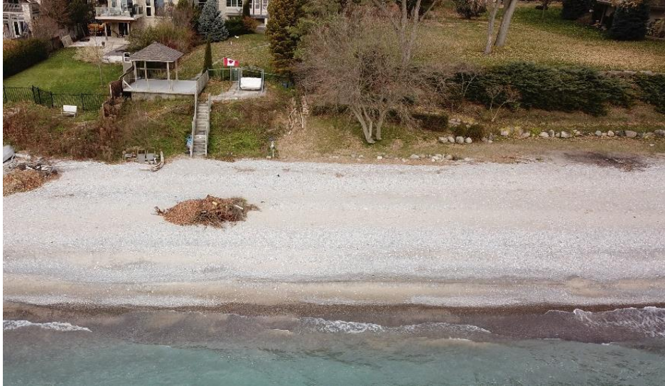
Central Section of Cove Road: Dynamic Beach Backed by Bluff - Photo courtesy of SJL Engineering (Nov. 2018)
