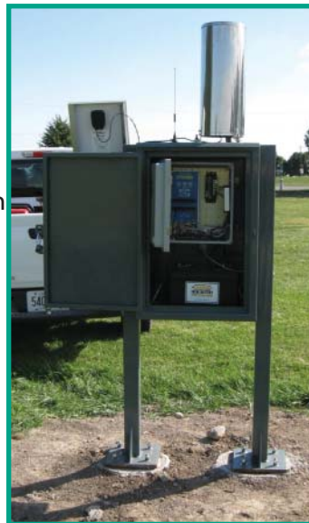
Precipitation water monitoring station.
