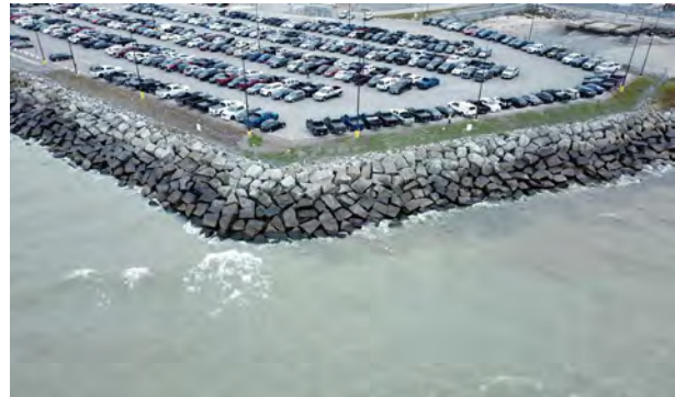
Shore Protection fronting Darlington Nuclear Power Plant
