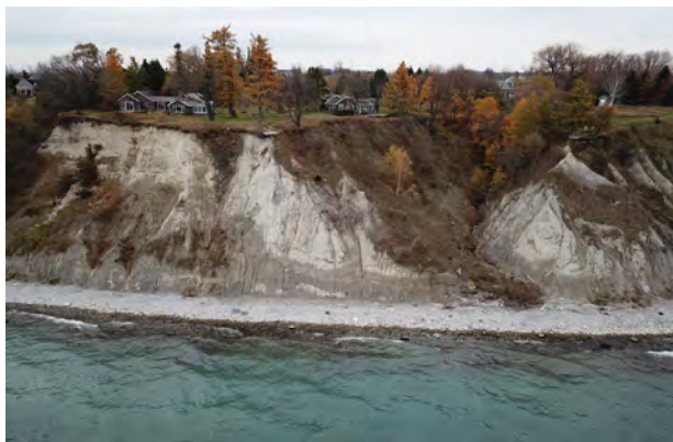
Eroding Bluffs at Bond Head
