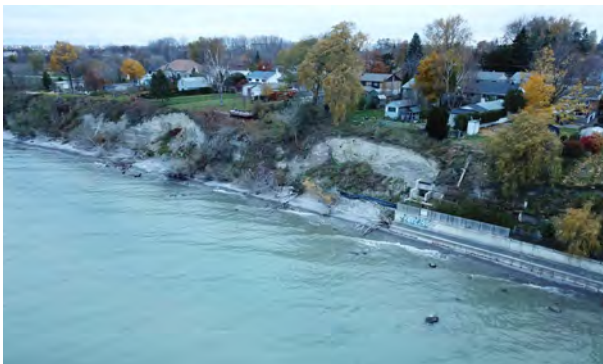
Eroding Bluff at Stone Street, Oshawa
