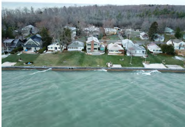
Concrete Seawalls, Presqu’ile Backside
