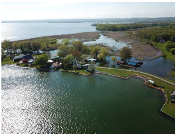
Flood Prone Properties, Evergreen Lane (May 2019)
