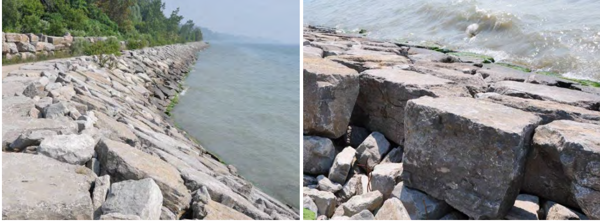
Figure 7.1 Sample armour stone revetments on Lake Ontario
