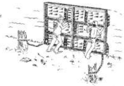
Figure 8: Flipping raft section into water.
