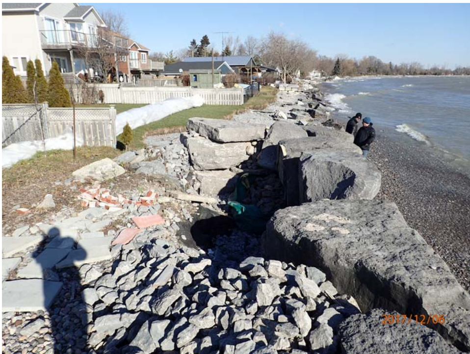
Figure 2.4: Armourstone protection at Cedar Crest Beach Road
